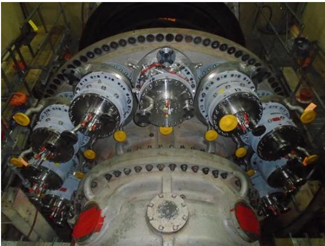
Figure 15. FlameSheet™ combustor configuration (before fuel delivery piping installation) of latest fleet additions
